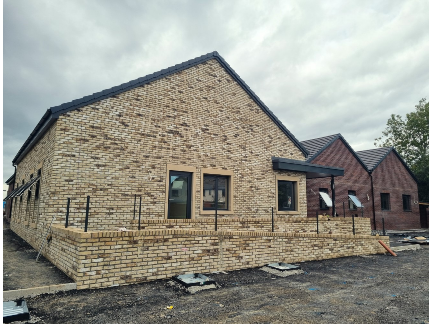
Limetree, front entrance; new build site, September 2023
